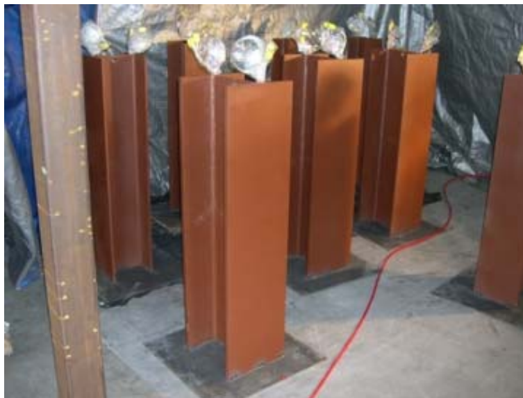
Columns ready to spray
