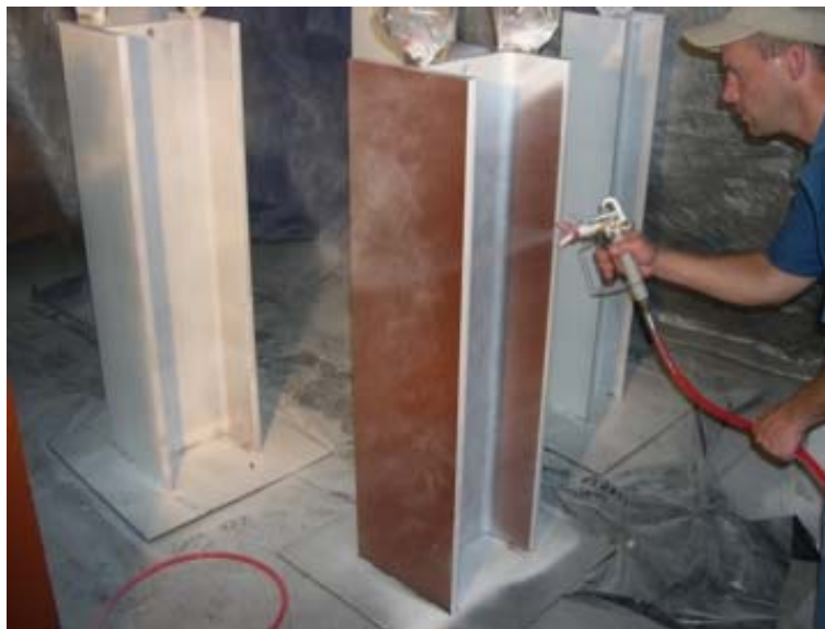
Applying the coating
