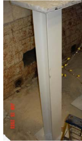
#8: Column in furnace.
