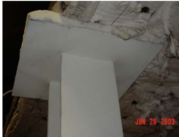
#10: Top of column in furnace.
