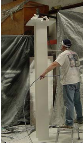
#7: Spraying the column.
