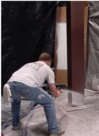
#5: Spraying the W10X49 column.
