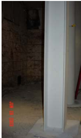
#9: Column in furnace.
