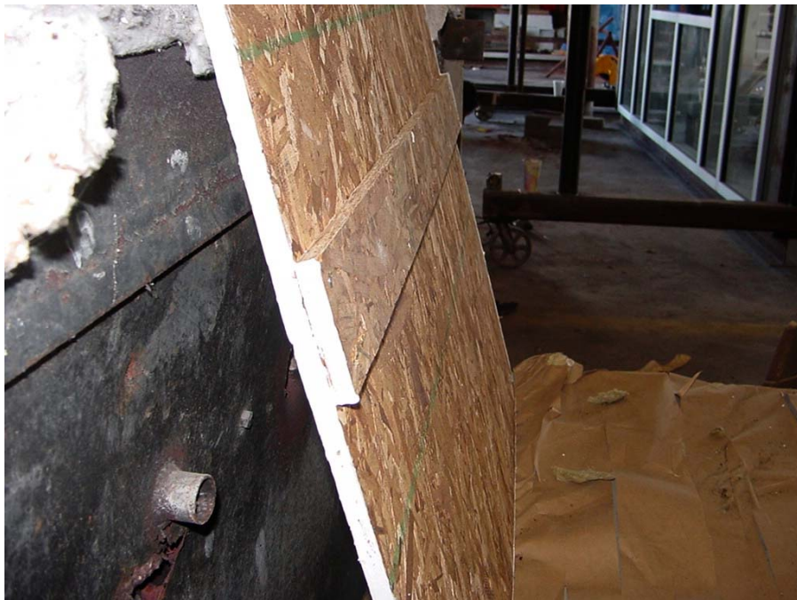
End view showing surface spline
